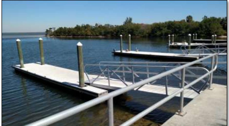
This project consisted of replacing two old floating flock, wood piles and gangways at the existing West boat ramp. The project included new security lighting around the existing boat ramps, walkways and existing restrooms.
