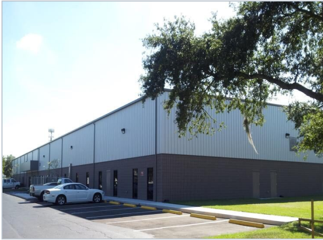
MAYER ELECTRIC, TAMPA
