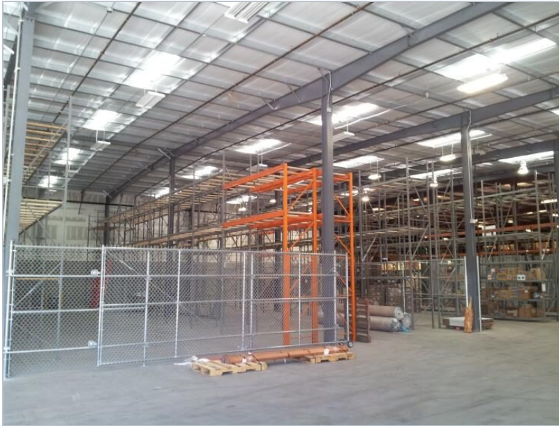
MAYER ELECTRIC · TAMPA, FL
